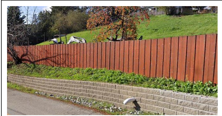
Lower parcel area, viewed from Glen Haven Road.
